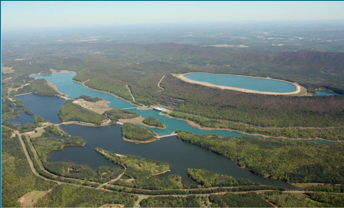
1095-MW Rocky Mountain Pumped Storage Project
